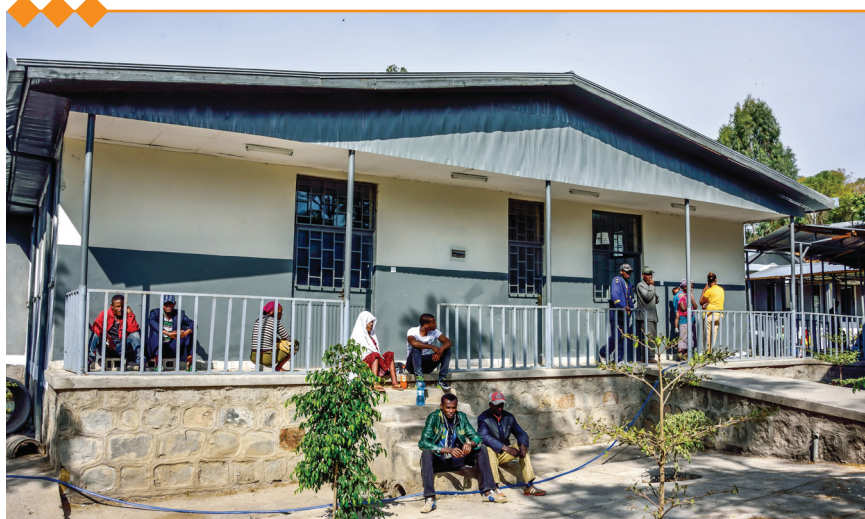
Bishoftu Hospital used retained revenue for several facility improvements, including the construction of a new 80-bed wing. The expansion doubles the hospital's admission capacity, improves patient flow, and increases service utilization.
