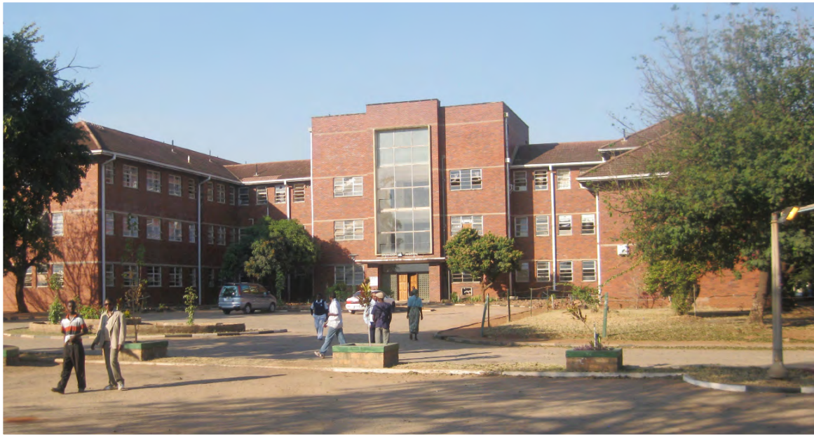
Second Level Hospital
